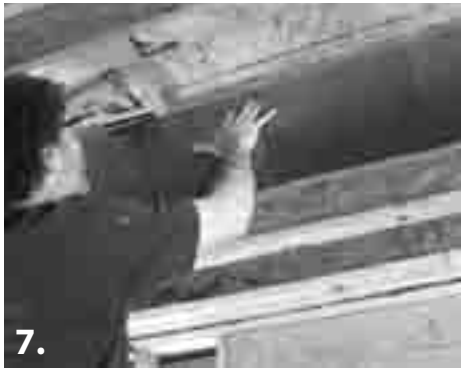
7. Continue stapling the mat mesh at 2" below the sub-floor, every 4" to 6". Then remove the nail at the end that held it up.
