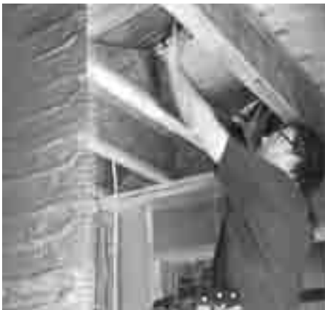
Test fit the mat between the joists before stapling the mat to the joists.
