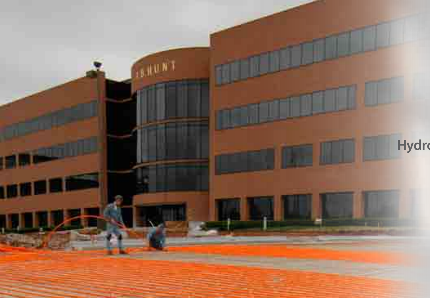
Brick Paver: Onix tubing embedded in sand beneath brick pavers.
